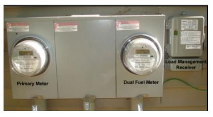
Double meter sockets are available for purchase from Jackson Electric Cooperative. It is the member's responsibility to contact Jackson Electric Cooperative to have the dual fuel load management receiver installed after all the wiring to the meter socket is complete.
