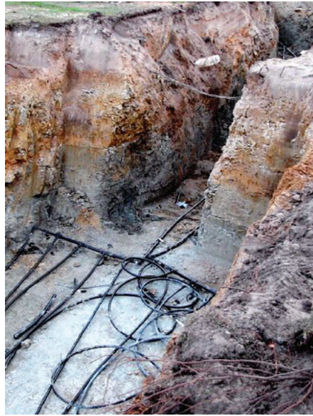
Left: In a closed-loop system, a pipe is laid in a trench that is typically six to eight feet deep. Fluid circulates through the piping, taking advantage of the earth's underground temperature. Right: You'll need about 400 to 500 feet of space for a horizontal, closed-loop system to be installed.
