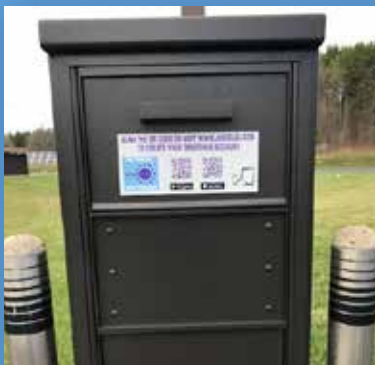
Secured payment drop box is located at Jackson Electric’s headquarters.
